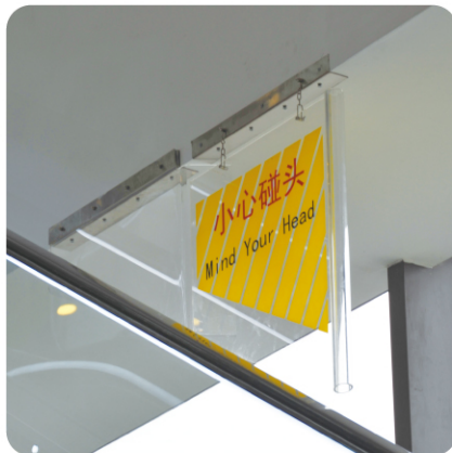
Vertical protective apron Prevent people from being caught at the included angle, causing personal injury (provided by customers)
